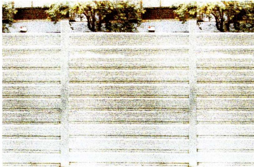
**CARACTERISTICAS :** PILAR : GALVANIZADO, ALTURA = 2,40 ml.
